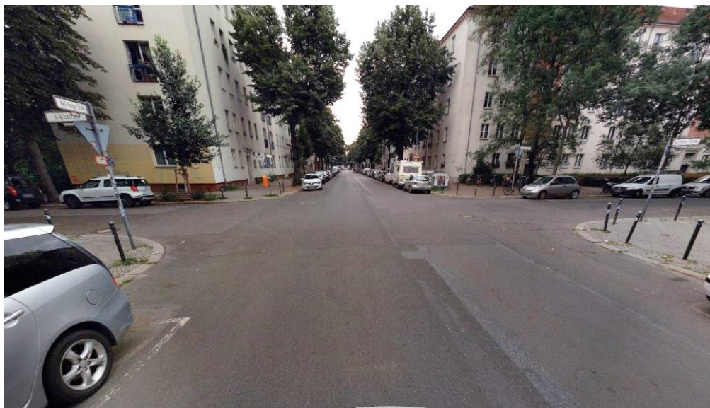
Bestand, Quelle: Infra3D
