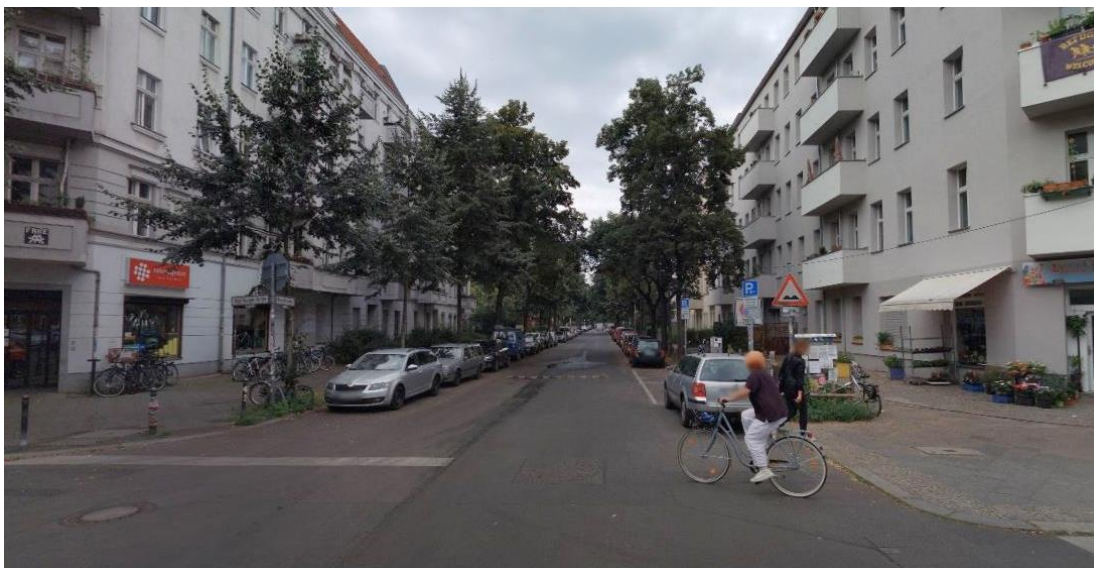
Bestand, Quelle: Infra3D
