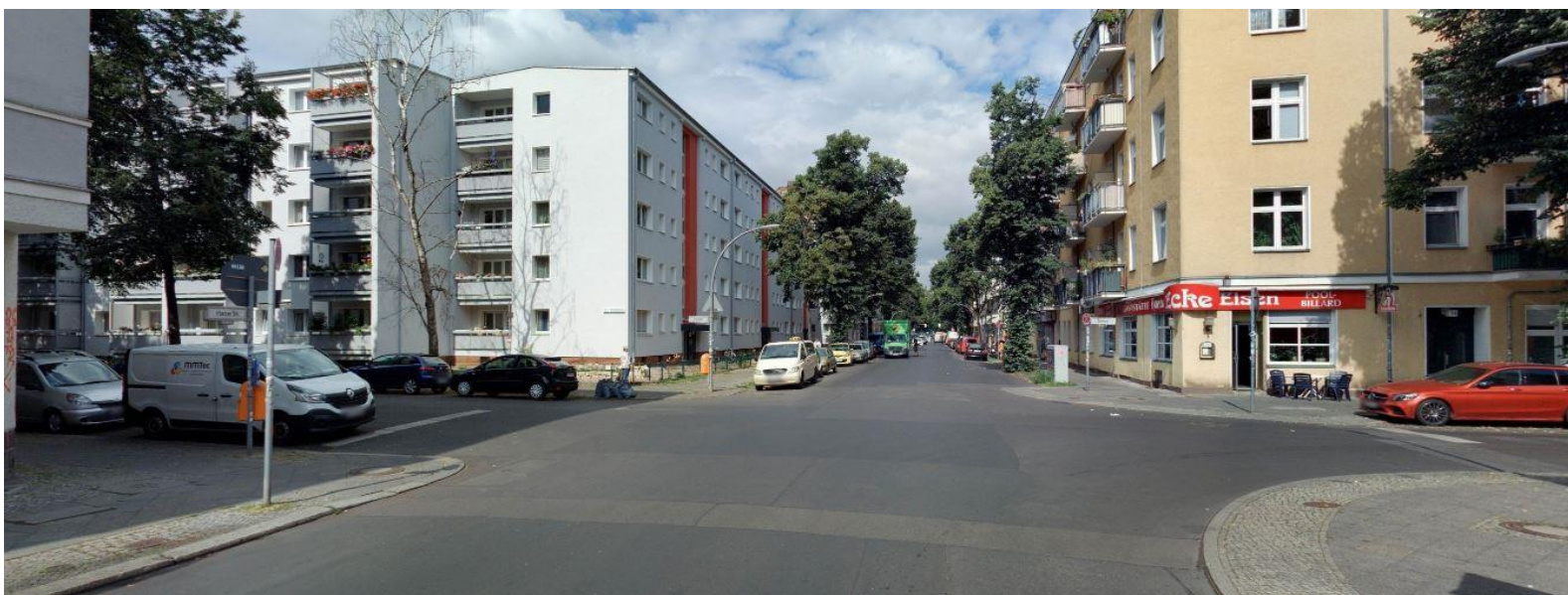
Bestand, Quelle: Infra3D
