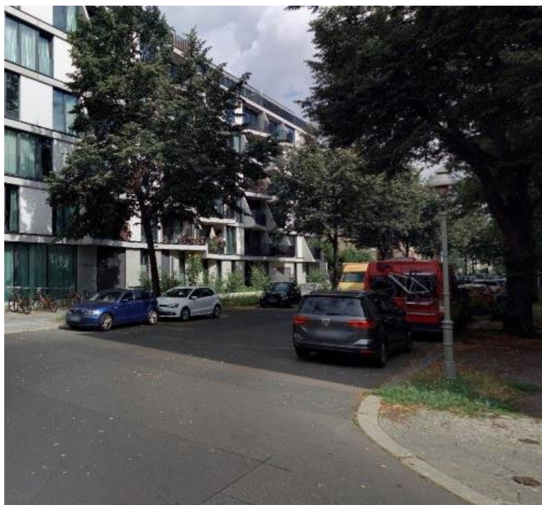
Bestand, Quelle: Infra3D
