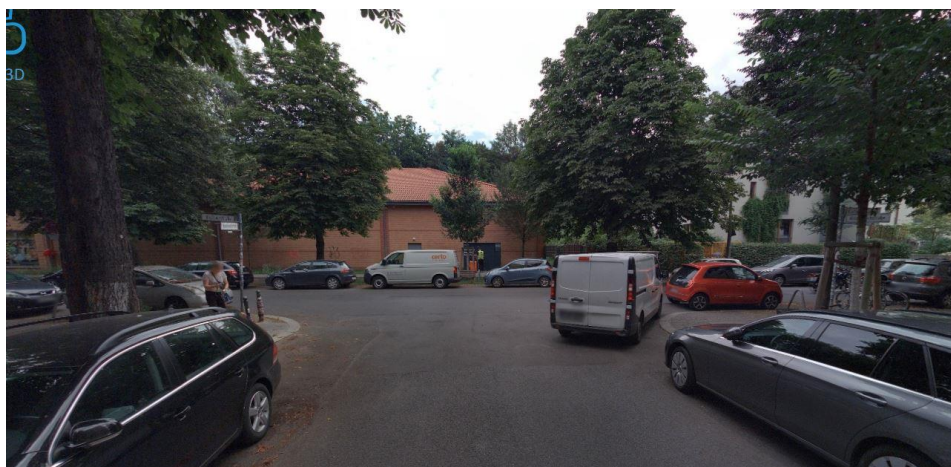
Bestand, Quelle: Infra3D
