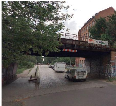
Bestand, Quelle: Infra3D
