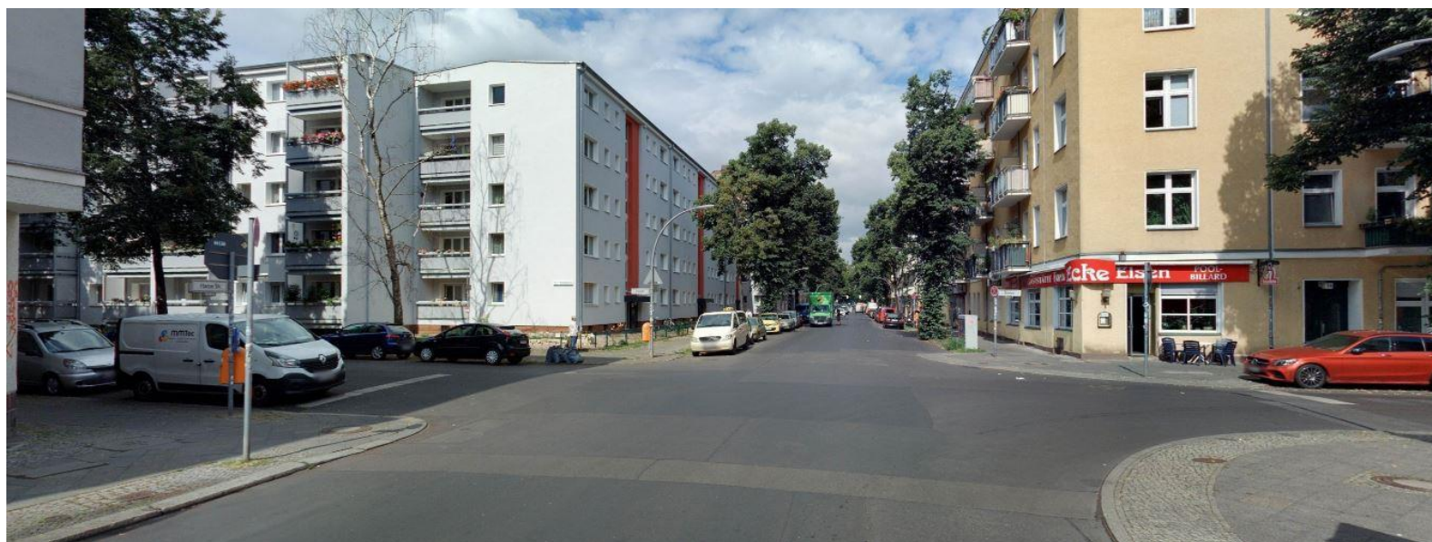
Bestand, Quelle: Infra3D
